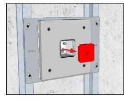
**3.** Remove the finishing guard from the fixture opening.
